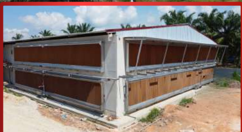
Pad Cooling System
