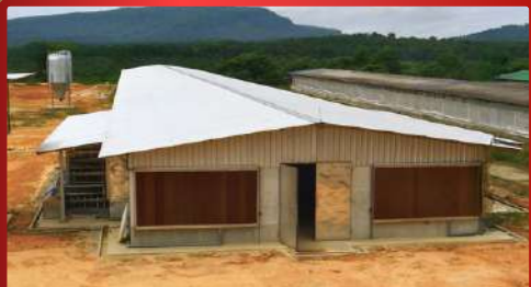
Pad Cooling System
